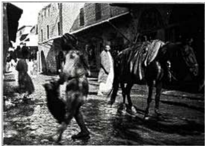
Hama's street sprinkler
