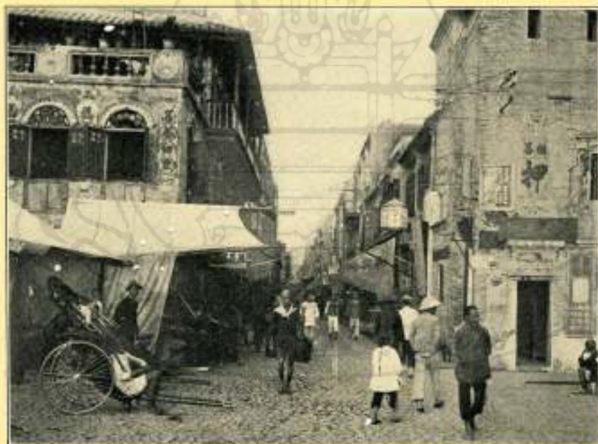
THE BUILDINGS IN HONG KONG (TOP) AND MACAO (BOTTOM) ARE OF MASONRY FOR THE MOST PART, NOT OF WOOD AS IN OTHER CHINESE CITIES, AND MOST OF THEM HAVE UPPER STOREYS (See p. 216)
