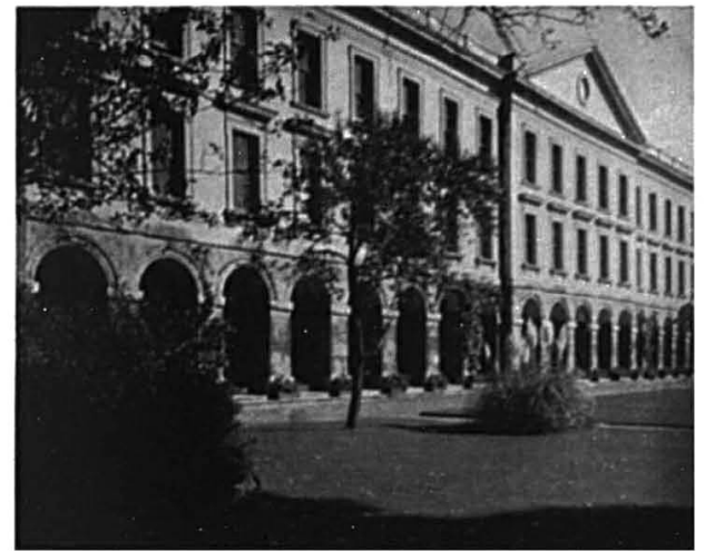
85 Magdalen : the New Building
