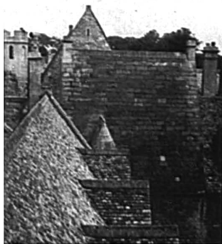
11 Mediæval Roofs at Merton
