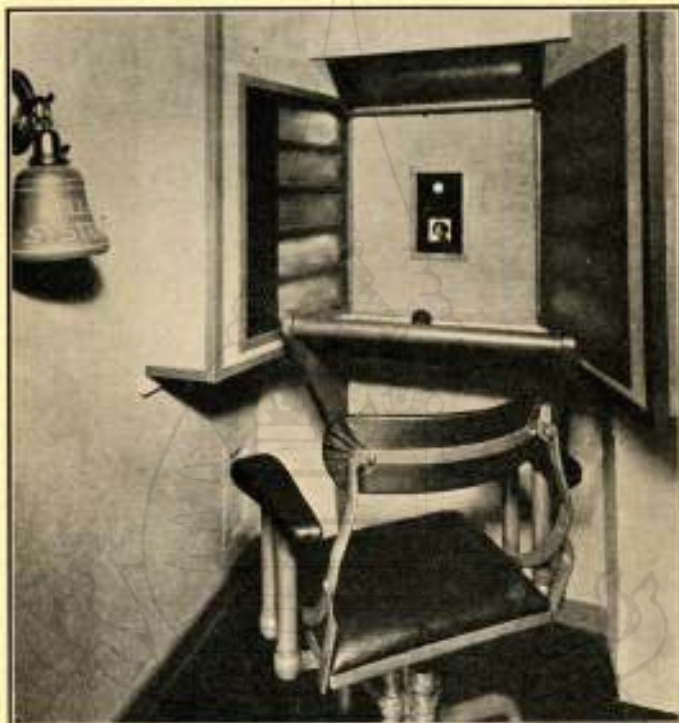
FIG. 13.—The booth used in the two-way wire television demonstration. The scanning light is projected to the subject just above the reproduction. The photoelectric cells are at each side and above the subject.
