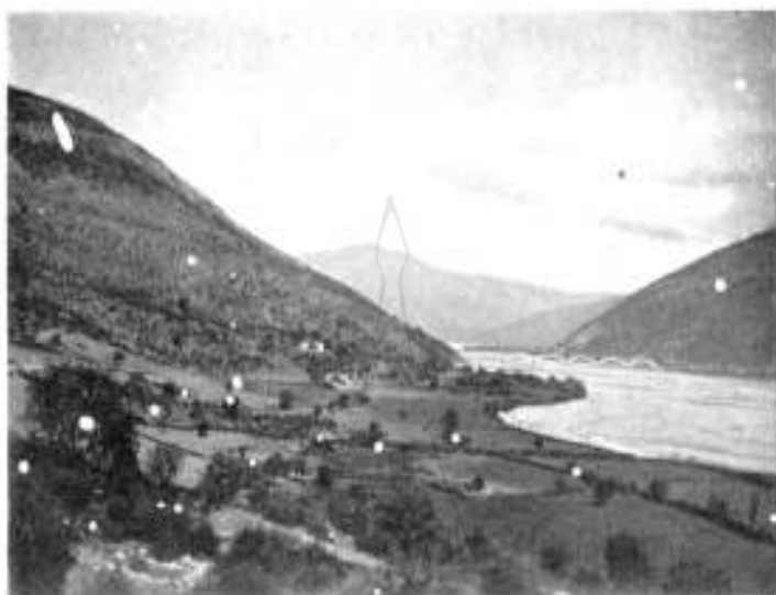
THE MATH RIVER AND THE NEW AHMED ZOGË BRIDGE
