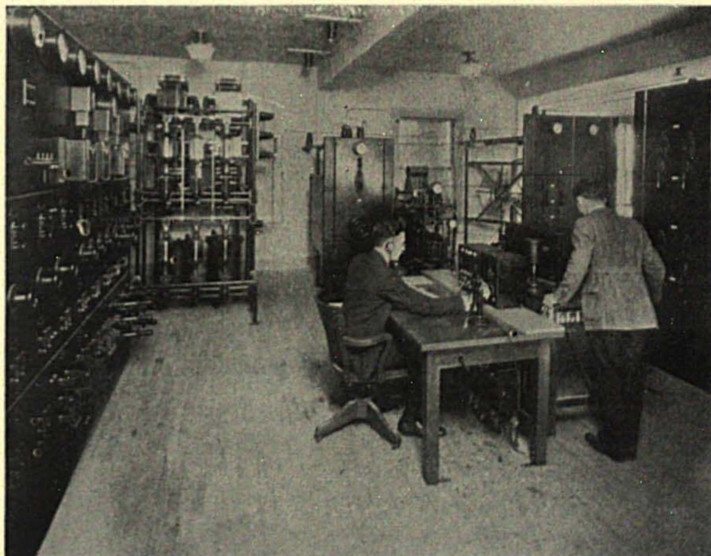
Fig. 237 Power Control Room, KGO, Oakland, Calif.
