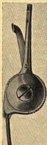
Fig. 9. - BRAKE LEVER FOR WINDMILL-DRIVEN COMPRESSORS
