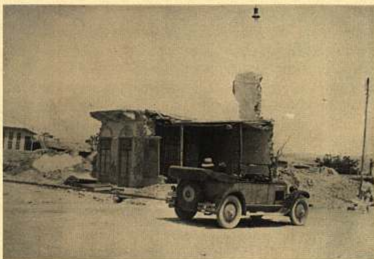
MODERN CORINTH IN RUINS FROM AN EARTHQUAKE
