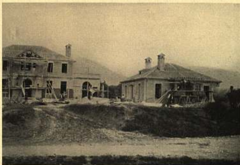
NEW GOVERNMENT-OWNED LEGATION BUILDINGS AT TIRANA
