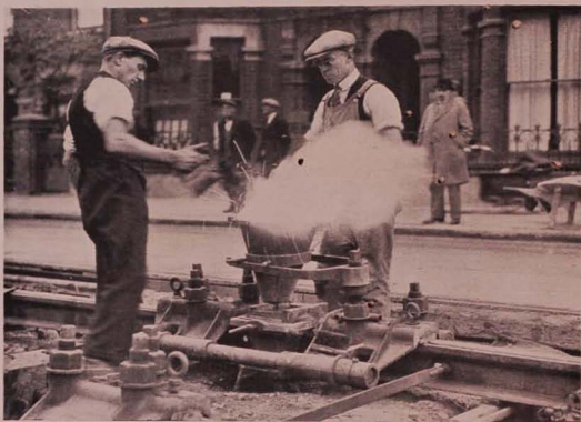
FIG. 1.—Tram-rail Welding by Thermit Process. (Courtesy, Messrs. Murex, Ltd., Rainham, Essex.)
