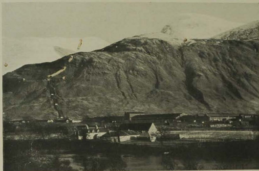
FIG. 57.—General View of the Lochaber Works of Messrs. The British Aluminium Co., Ltd., showing Pipe Line in Background to supply the Works with Water Power.
