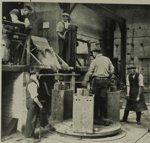
FIG. 49.—Electric Induction Furnace for the Manufacture of Stainless and Special Steels.
