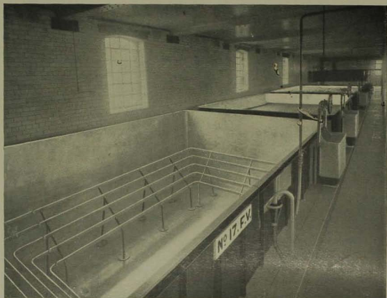
FIG. 60.—Aluminium Fermenting Vessels used in a Bolton Brewery. They are made of Thick Sheets of Aluminium welded together so as to provide a dead smooth interior surface, the exterior being reinforced with Mild Steel Stanchions.
