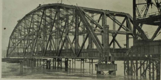
FIG. 51.—The Quebec Bridge. The Cantilever Piers are 1,800 feet apart. Its construction was made possible by the use of Stainless Steel (i.e., containing Nickel and Chromium).
